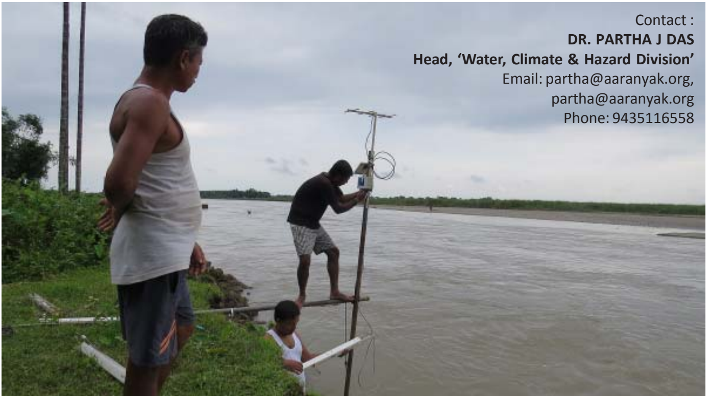
Installation work of the Community Based Flood Early Warning System(CB-FEWS) in progress in DijuChapori on the bank of the river Ranganadi, Lakhimpur District on July 19, 2016. Photo: Partha Jyoti Das
